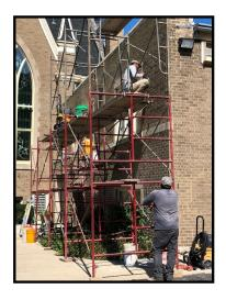
The masons repaired several bays on the church and both the replacement brick and the mortar match well.
